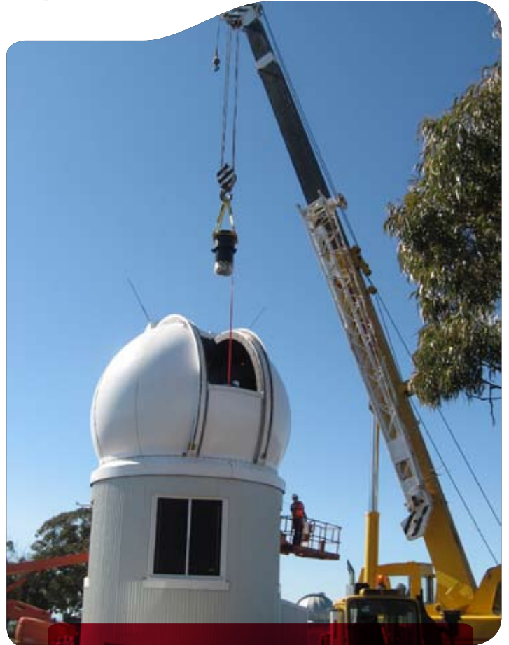
THE CORRECTOR LENS ASSEMBLY IS LOWERED INTO THE SKYMAPPER TELESCOPE.
